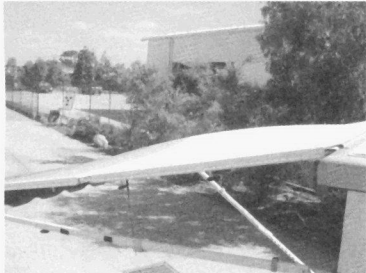
SHOWS CURVED ROOF RAFTER IN POSITION
